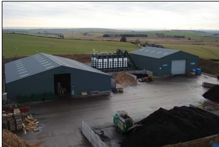
The VCU™ facility at Keenan Recycling, New Deer
