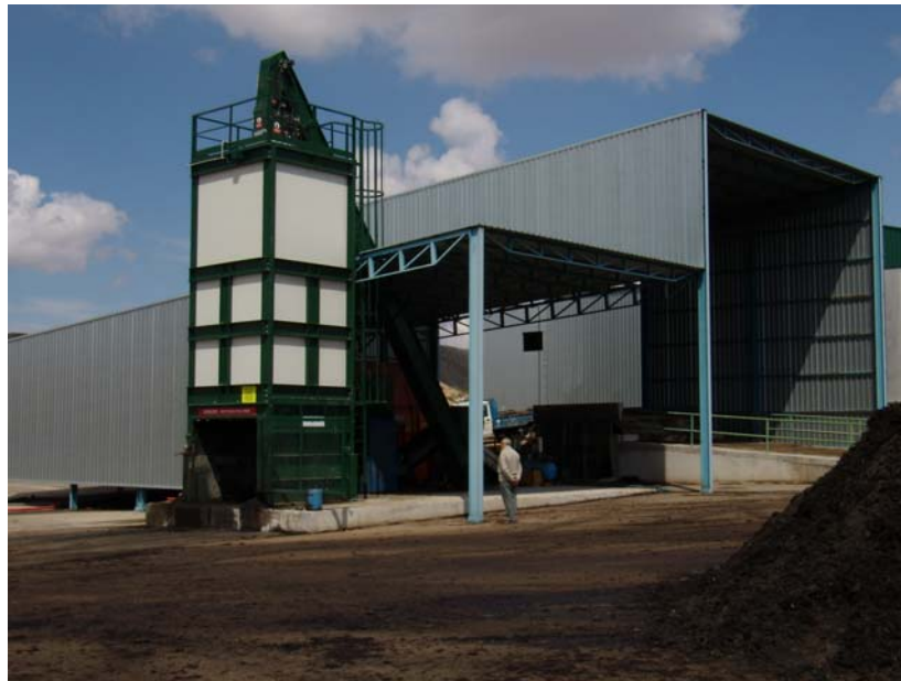
The existing VCU Installation at Sana SL, which will be expanded to meet increasing demand for extra capacity
